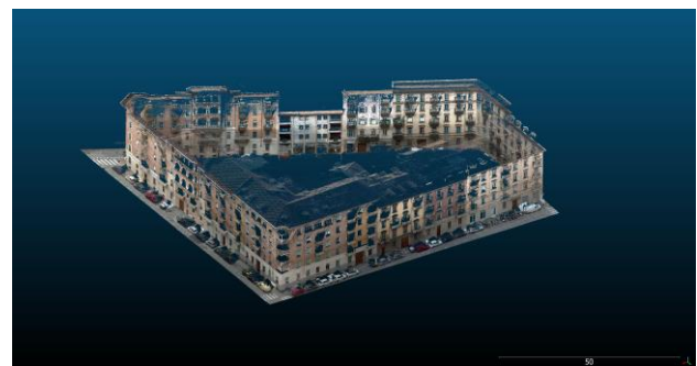
Figure 3. Point cloud of the test site resulted from the acquisition from aerial LiDAR.
