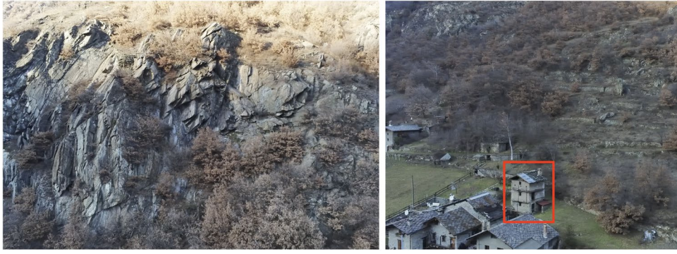
Fig. 2 View of the source area (left) and the deposit (right) where the elements at risk are located
