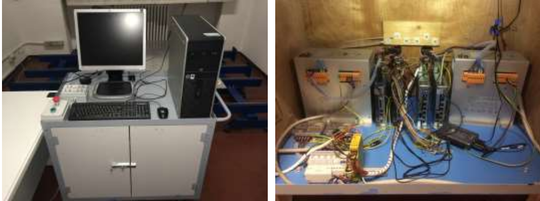
Figure 9. Control panel and workstation and electronic devices inside the control panel.
