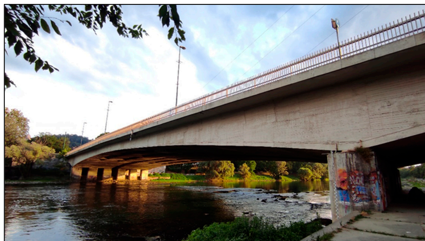
Figure 8. Close-up view of the Corso Regina Margherita Bridge (V1-T), which is the subject of this and other ongoing research.
