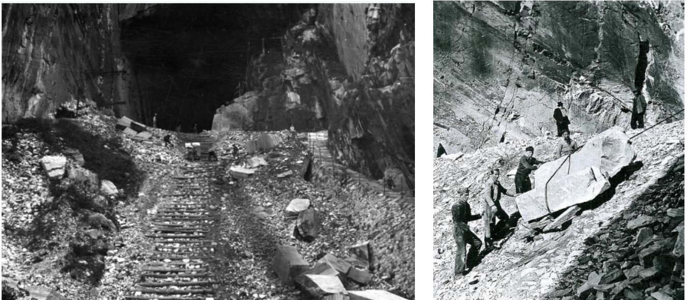
Figure 6. Cava Madre of Candoglia. Ancient road ("via di lizza") equipped to allow the transport of blocks (left) and the "lizzatura" phase using ropes and wooden planks.
