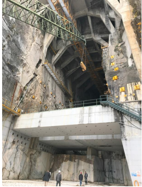
Figure 3. Detail of the entrance area of the Cava Madre (left) and detail of the three imposing strut-beams in reinforced concrete built at the beginning of the 2000s to counteract the lateral thrusts of the walls.
