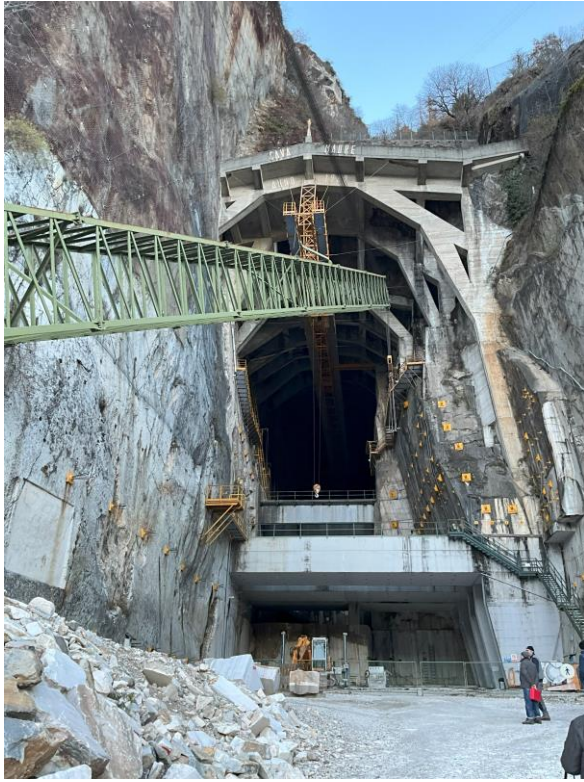
Figure 3. Detail of the entrance area of the Cava Madre (left) and detail of the three imposing strut-beams in reinforced concrete built at the beginning of the 2000s to counteract the lateral thrusts of the walls.
