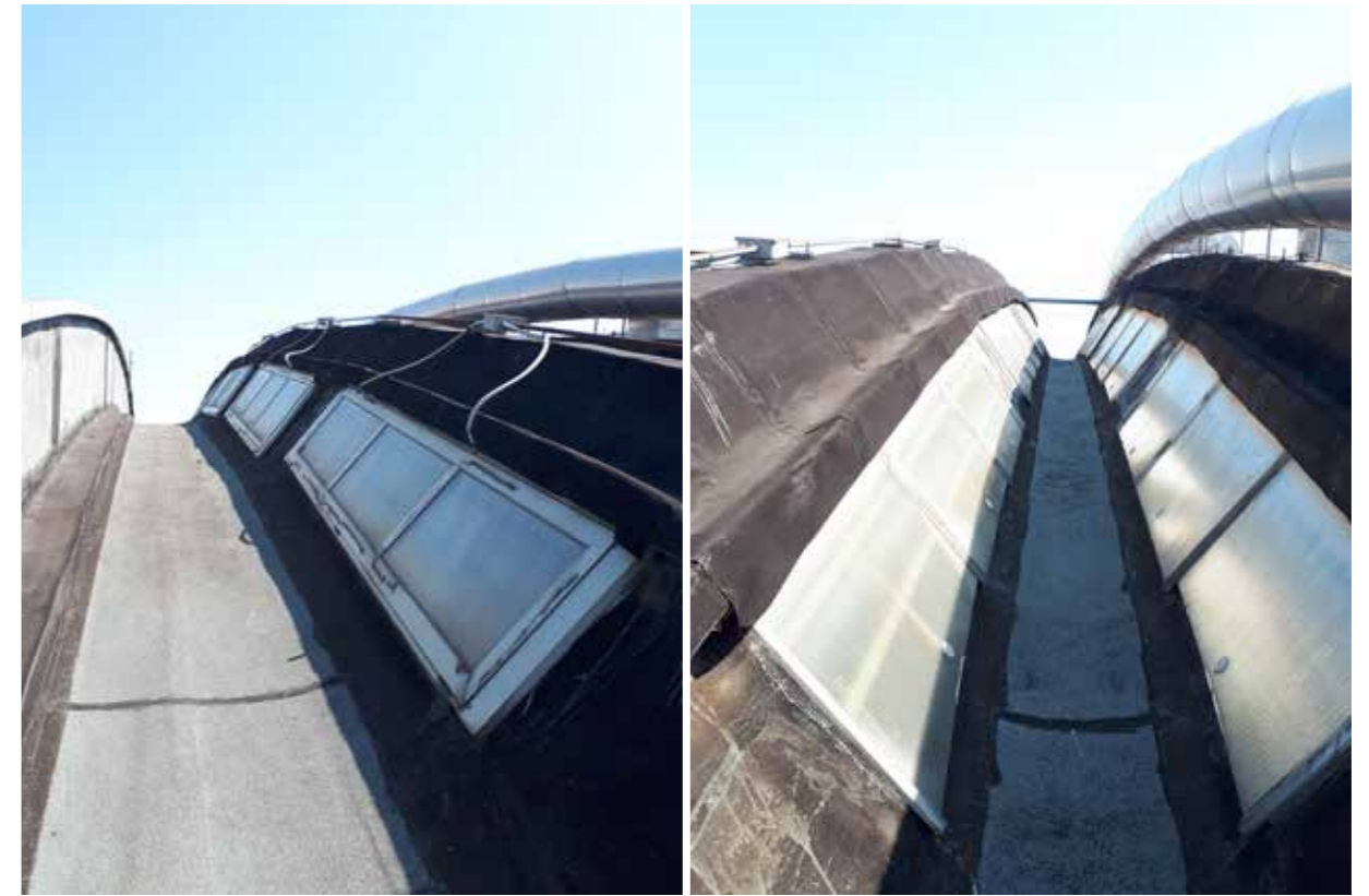
3c 5.8: Different types of skylights in the roof of Hall B, with an automatic opening mechanism that requires a larger frame and fixed openings
