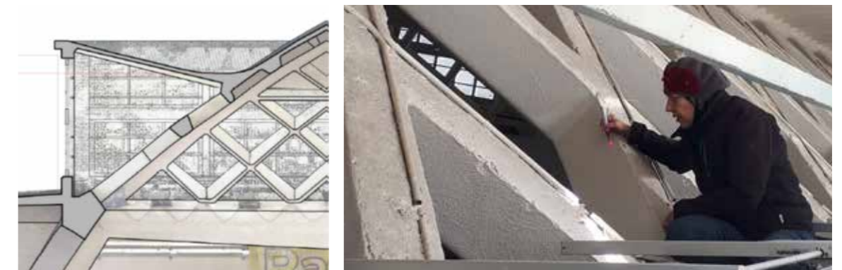
3c 5.4: A view of the same construction detail using the drawing with the overlapped orthophoto and a phase of the topographic measurement to assess the intrados-extrados relationship.
