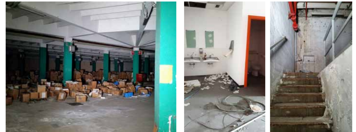
3a 3.4. a, b, c: For underground environments, it was necessary to use traditional 3D scans, but in general, all the service areas and stairs were detected by means of mobile scans from hand-held scanners.
