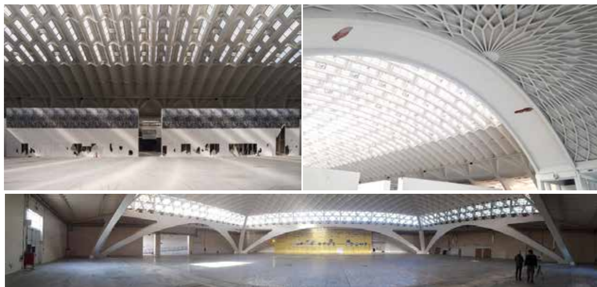
3a 3.3.a, b, c: Interior environments object of the 3D detailed survey methods using traditional laser scanning techniques, a hybrid technique from the Swift mobile system and terrestrial photogrammetry for the structural elements and related diagnosis.
