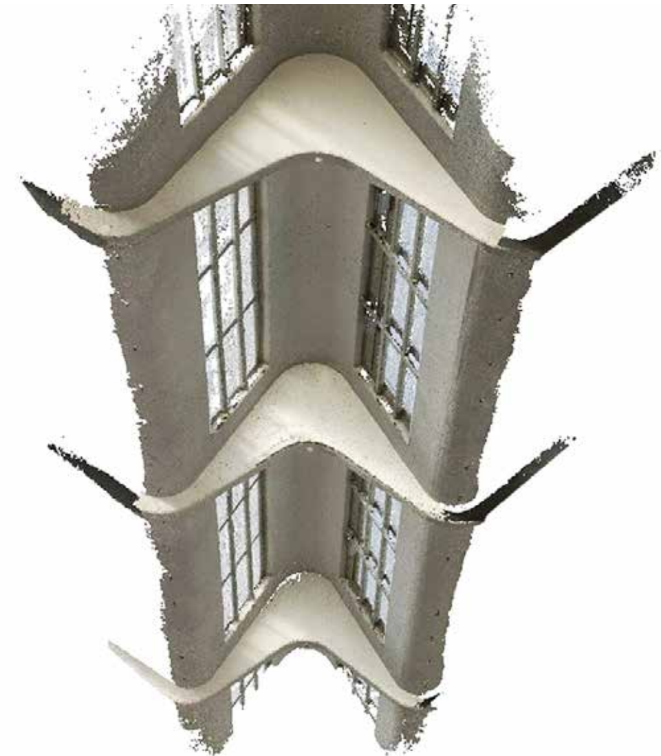
3a 9.7: Project drawings of the wave elements of Hall B, and photogrammetric reconstruction of a module of the vault.
