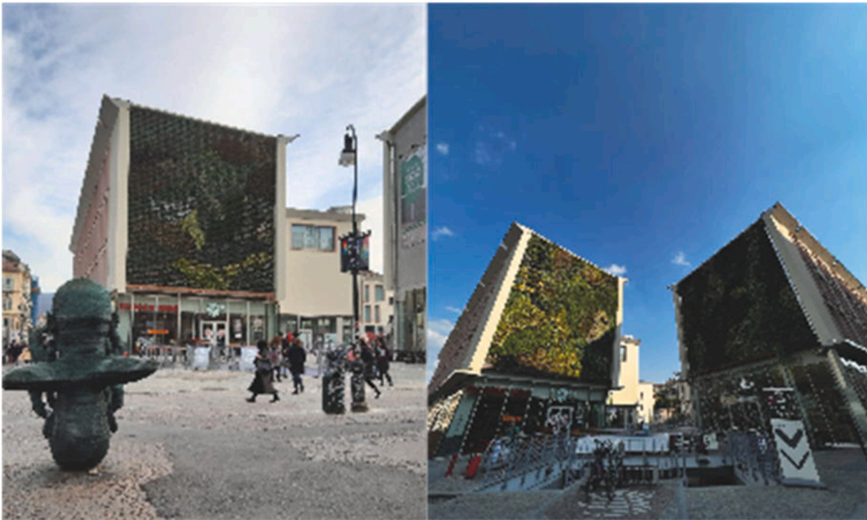
Fig. 3. Green walls in CAM.
