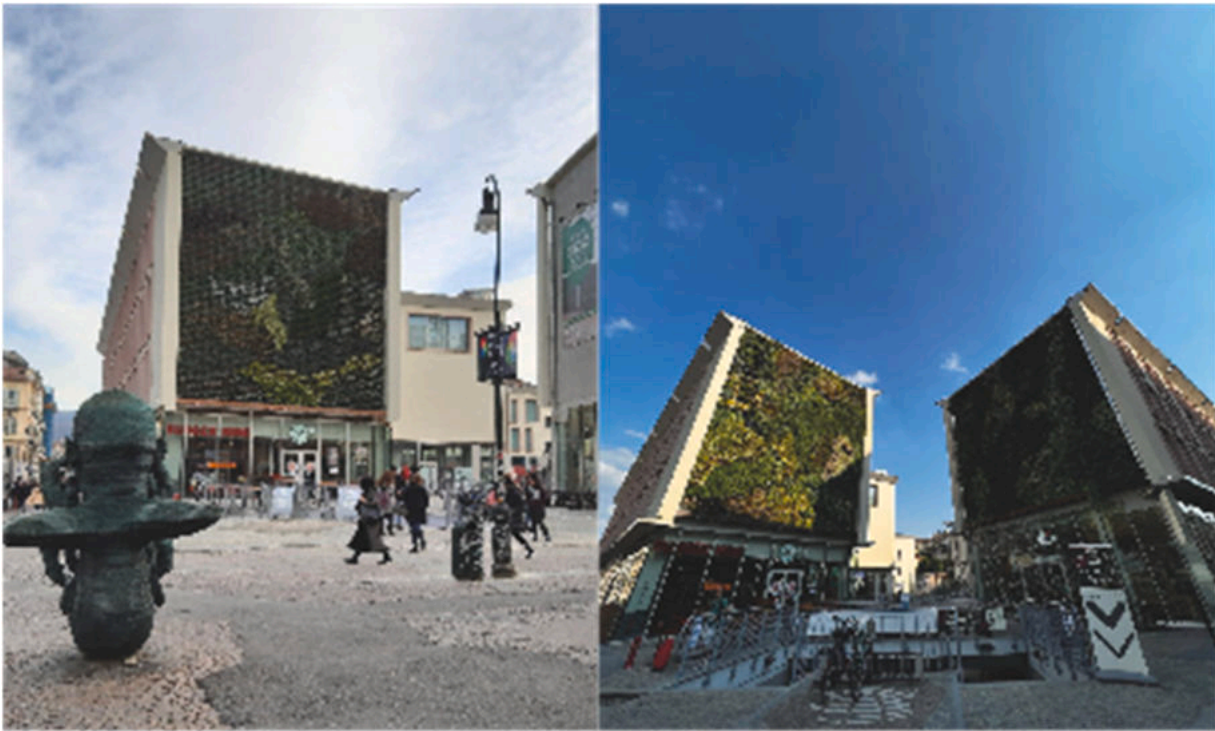
Fig. 3. Green walls in CAM.
