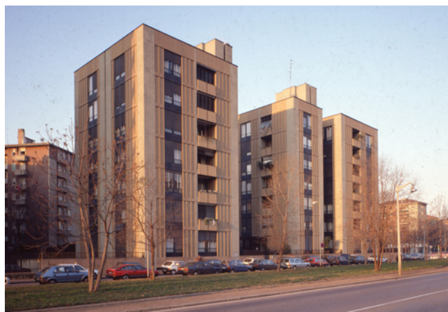
Figure 8. The building complex in via Palmanova, Milan, 1962–67. (CASVA, AA archive collection).
