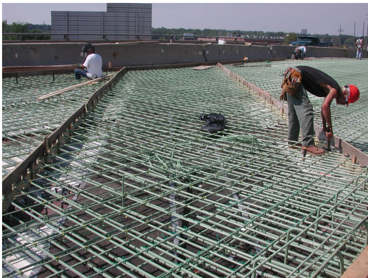
Fig. 4 Traditional construction site: The placing of reinforcements
