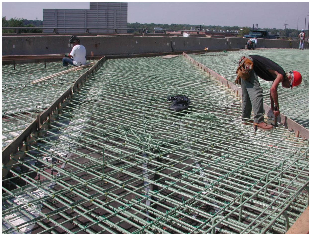
Fig. 4 Traditional construction site: The placing of reinforcements
