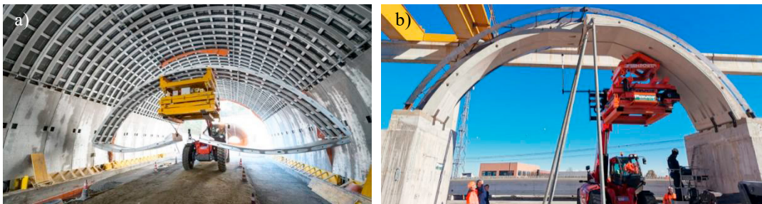
Fig. 9 a) Relining by liner plates - Pilot application at “Castello” tunnel, b) “Poderuzzo” tunnel - Field test of pre-cast concrete shell implementation
