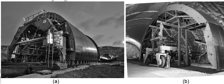
Figure 6.27 Self-reacting formwork (a) and turret-type formwork (b).
