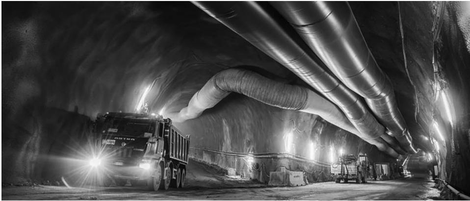
Figure 6.56 Ventilation ducts in the Mules adit.
