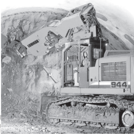
Figure 6.9 Example of an excavator working on a tunnel face and its operational area. (Courtesy of Liebherr.)
