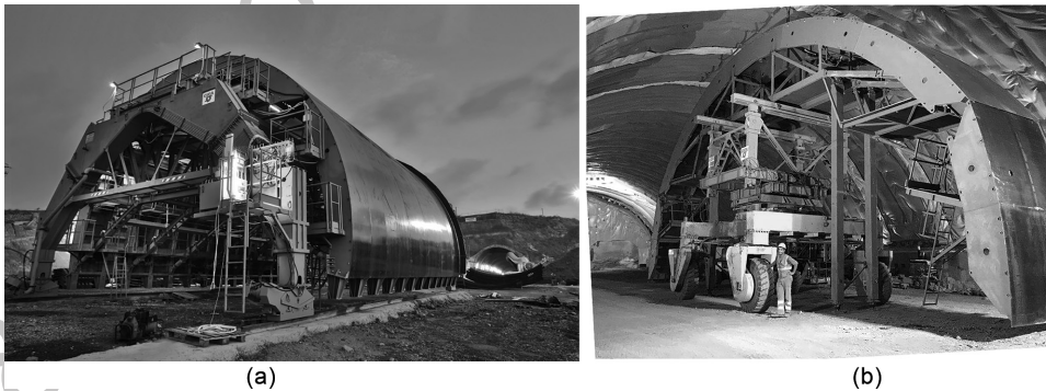
Figure 6.27 Self-reacting formwork (a) and turret-type formwork (b).
