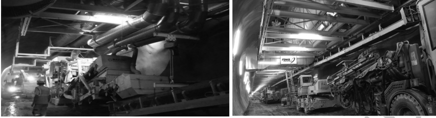
Figure 6.18 Telescopic ventilation platform for fresh air supply, allowing efficient suction ventilation of blasting fumes as well as increased working safety, thanks to free floor space for working and parking.
