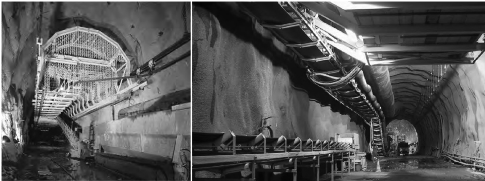
Figure 6.17 View of equipment from tunnel face; crusher and hanged conveyor belt.
