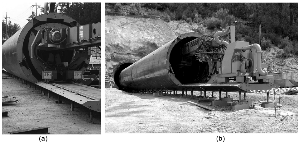
Figure 6.31 Full round formwork (a) and continuous casting full round formwork (b).
