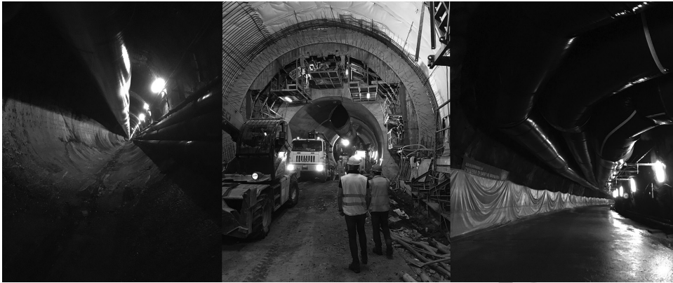
Figure 6.54 Ducts installation inside tunnel.
