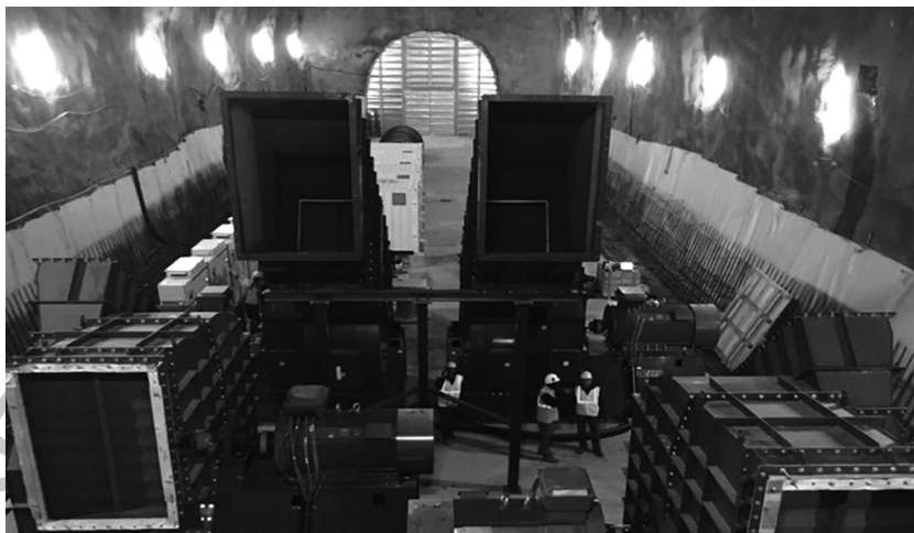
Figure 6.57 Centrifugal fans during installation.
