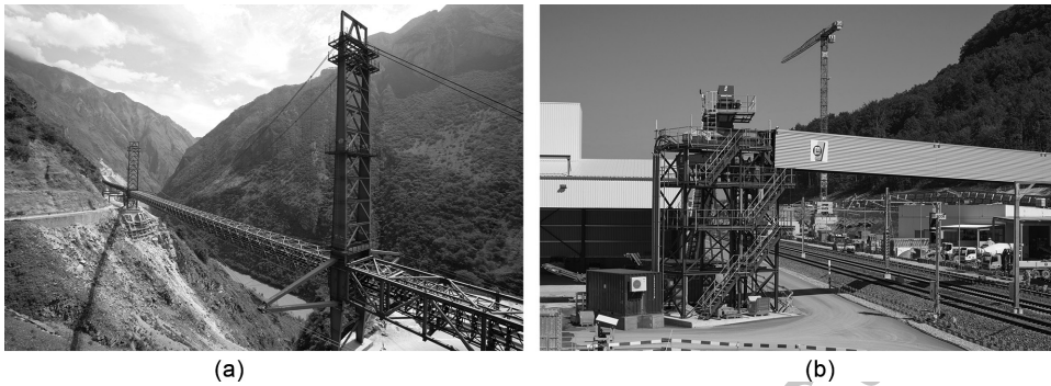
Figure 6.5 Belt conveyor over a gorge (a). Belt conveyor crossing railways and streets (b). (Courtesy of Marti Technik.)
