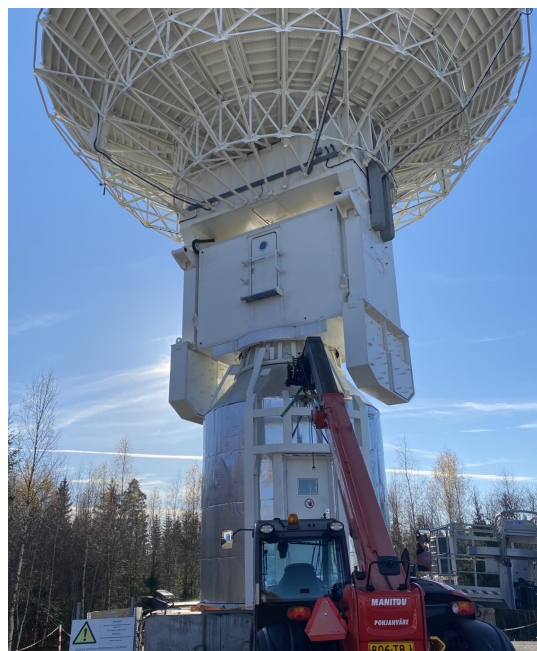
Fig. 2 Work on the telescope pedestal insulation (October 2022).
