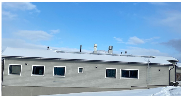
Fig. 3 New main building.
