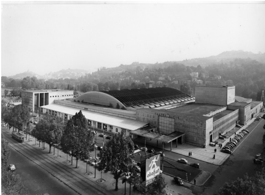
Fig. 1. Aerial view of the exhibition center Torino Esposizioni in 1954 (Archivio Storico Fiat).
