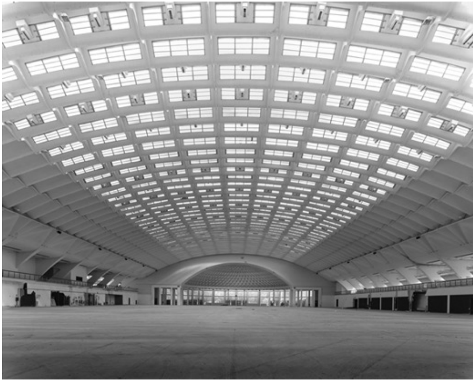
Fig. 5. Hall B, after the clearing and cleaning operations for the execution of the tests of the Getty Keeping It Modern project (courtesy of Fabio Oggero, 2022).
