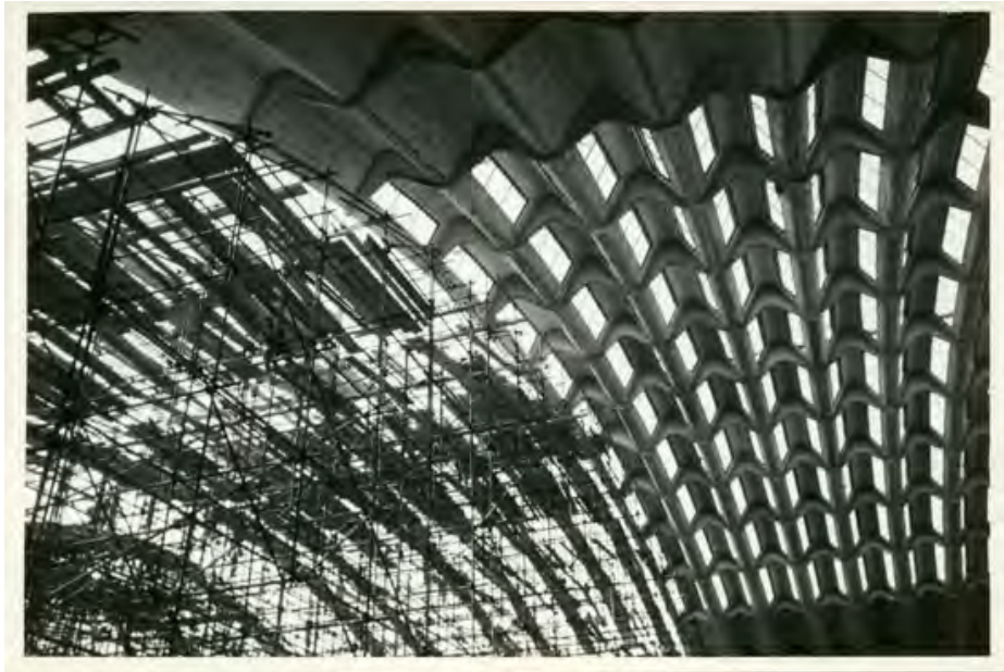
Fig. 4. This photo of the construction site shows the mobile scaffolding system used to build the vault (Archivio Privato Ravelli).
