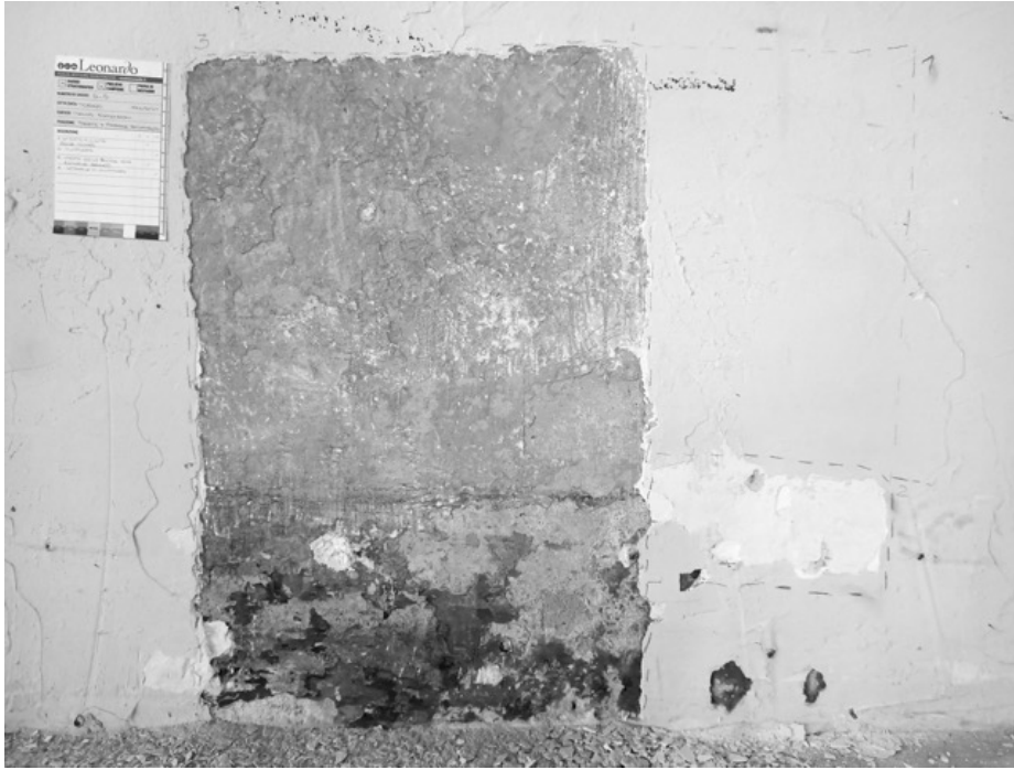
Fig. 6. The bichrome area between the beige wall and the brown plinth, visible in the lower areas of the walls of Hall C and the pillars of Hall B.
