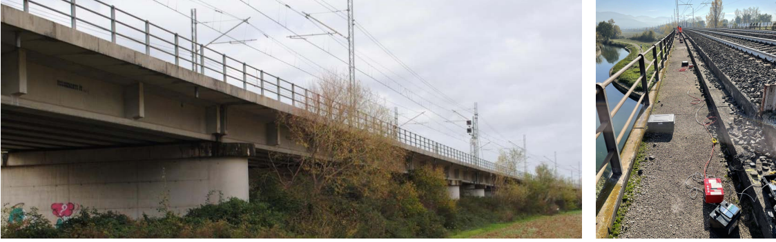
Figure 2.24: Orte-Falconara bridge case study: viaduct overview and ambient vibration testing.
