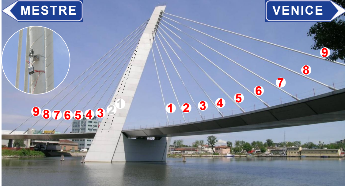
Figure 2.18: Marghera bridge case study: global overview.
