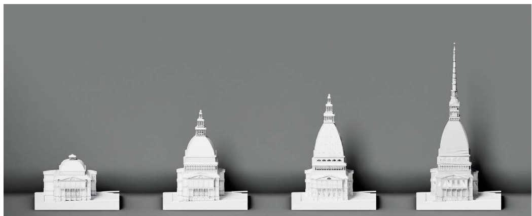
Different virtual configurations of the Mole Antonelliana in Turin by Alessandro Antonelli's various design proposals. Elaboration by L. Torresi.
