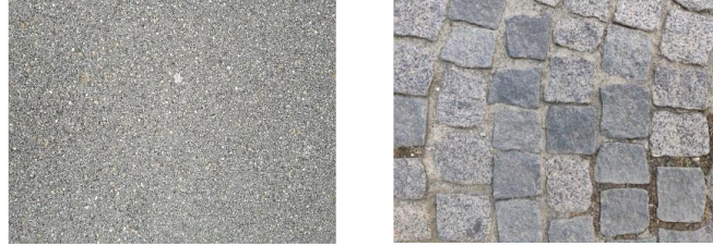
Fig. 2. Tested textures: asphalt (on the left) and pavé (on the right).
