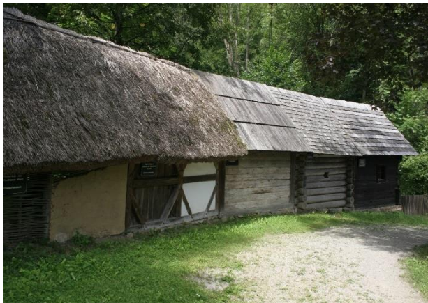
Figure 1. Different building technologies for same function and typology at Österreichisches Freilichtmuseum Stübing, Austria. Photo: A Bocco Guarneri, 2011.
