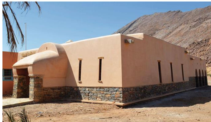
Figure 4. Exterior view of the Maison de la maternité, Tissint, Morocco, 2017. Credit: S Naji www.salimanaji.org/salima_naji/2017/08/
