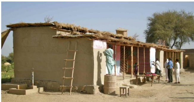
Figure 5. Flood response shelter designed by Yasmeen Lari, 2010. Credit: the Heritage Foundation of Pakistan.
