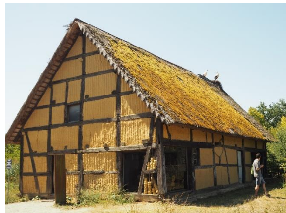
Figure 2. Rural house mostly built with agricultural material at Écomusée d’Alsace, Ungersheim, France. Photo: A Bocco Guarneri, 2020.
