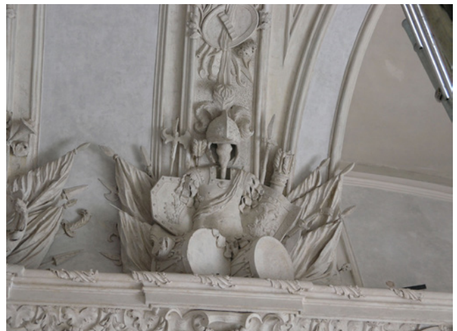
Figure 3. Royal palace of Venaria Reale and the detail of the stucco work by the Swiss artist Piscina (picture by the author, 2022).
