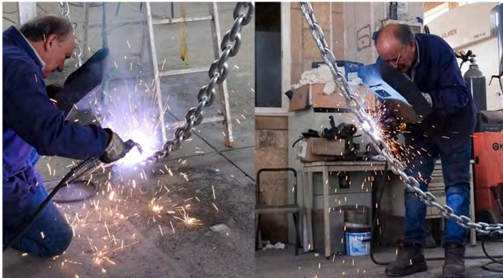
Fig. 4. The welding phase of the real scale arch.
