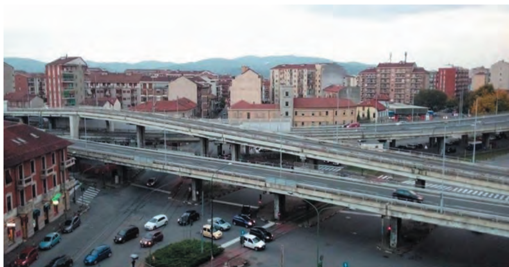
Figure 1. Corso Grosseto viaduct before the dismantling.
