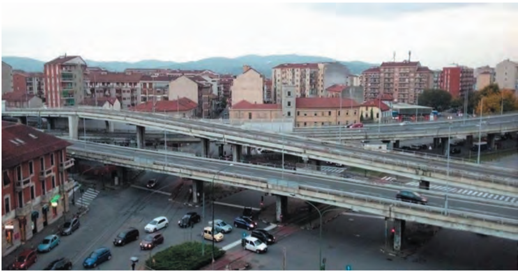
Figure 1. Corso Grosseto viaduct before the dismantling.
