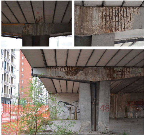
Figure 3. View of the bridge deck and details of the pier caps.
