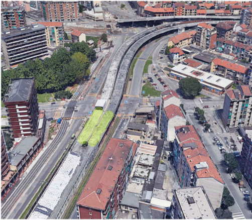
Figure 1. Aerial view of the Corso Grosseto viaduct.
