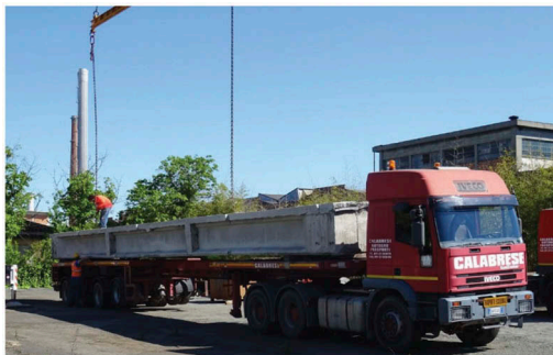
Figure 7. Beams moved by trucks to the testing site.
