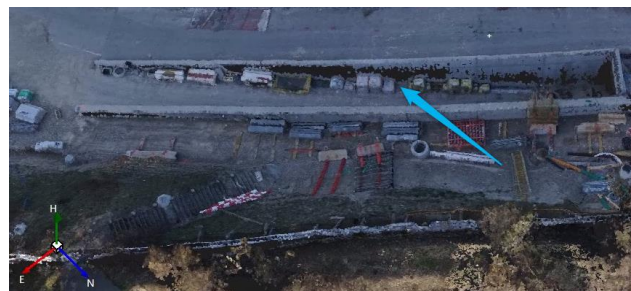
Figure 7. Example of missing data in a narrow driveway due to obstructions.
