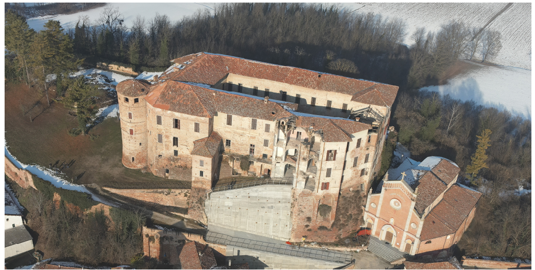
Figure 1. Frinco Castle from the UAS P1 sensor. Overview of the southwest side and the collapsed area.
