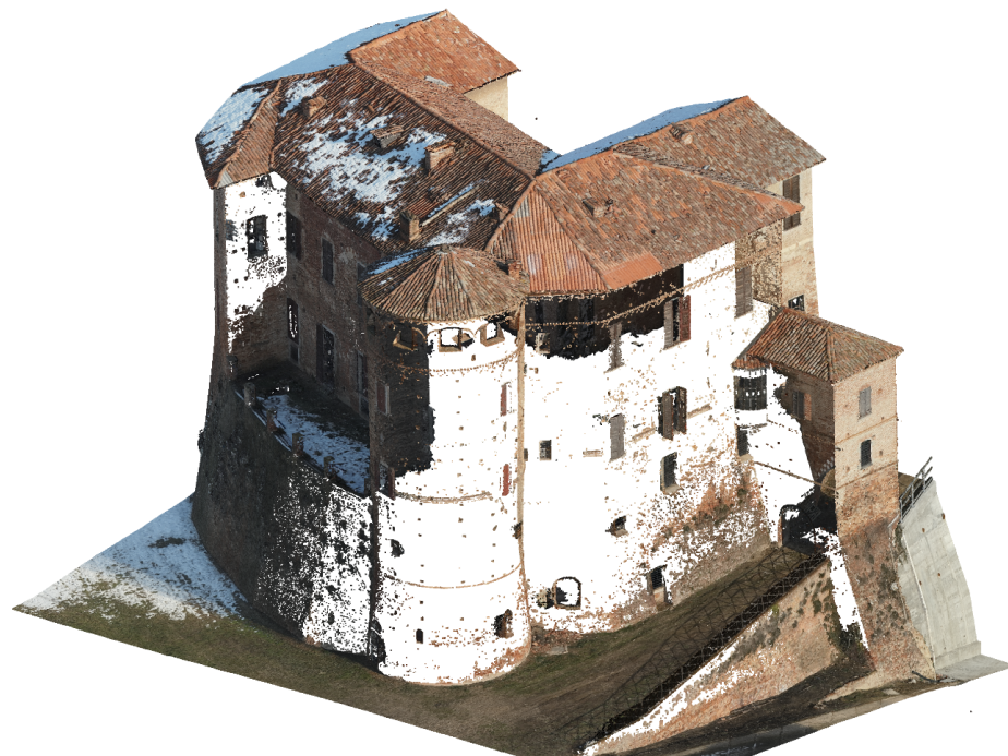
Figure 22. Photogrammetric point cloud of the selected points.
