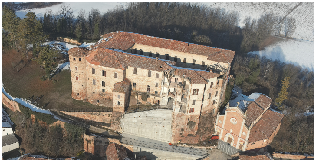
Figure 1. Frinco Castle from the UAS P1 sensor. Overview of the southwest side and the collapsed area.
