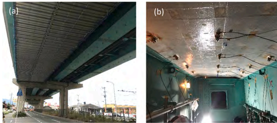
Fig. 13. (a) Tested highway bridge, (b) sensor arrangement for the measurement before repair.
