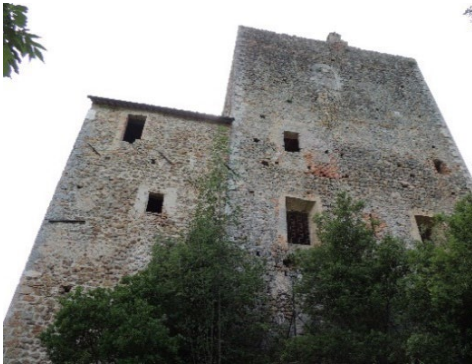
Fig. 4- The north façade of the summit area with the evident resting of the second-period tower to the left (CF2) on the older tower (CF1) to the right (photo by F. Fratini)
