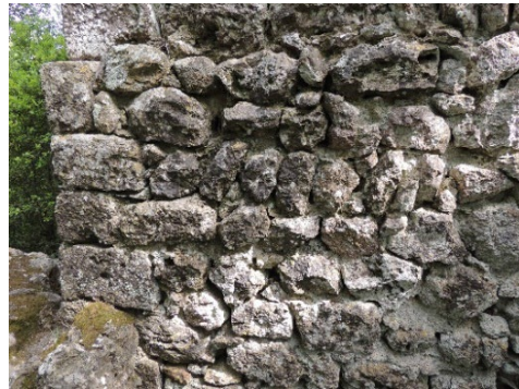
Fig. 5- Detail of the construction technique of Period 1 (photo by F. Fratini)
