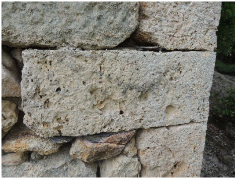
Fig. 7- Corner stones made of travertine (photo by F. Fratini)
