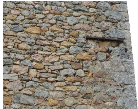
Fig. 10- Detail of the construction technique of Period 3 (photo by A. Arrighetti)
