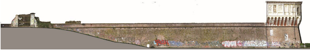
Fig. 3- Orthoimage of the whole wall (Elaboration: M. Russo)
