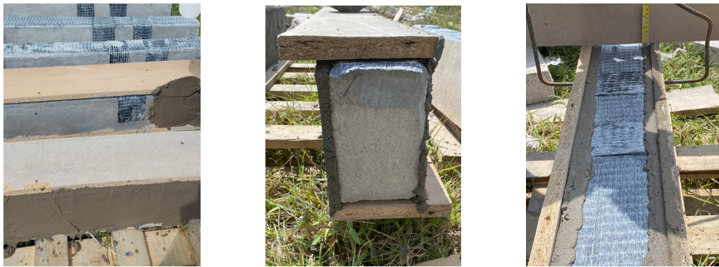
(a) Applying the mortar
