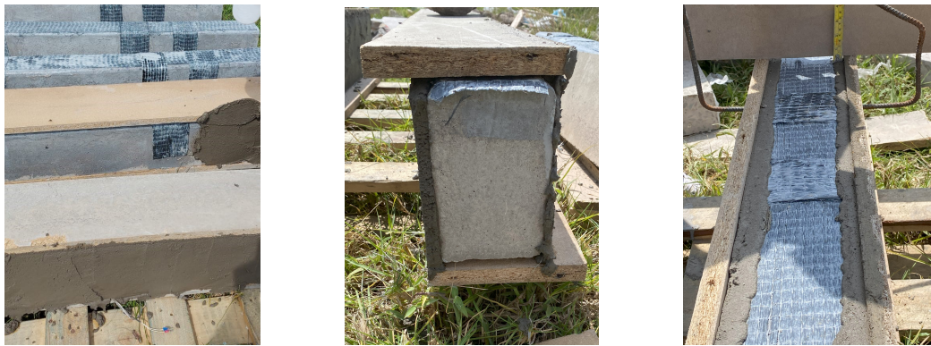
(a) Applying the mortar
