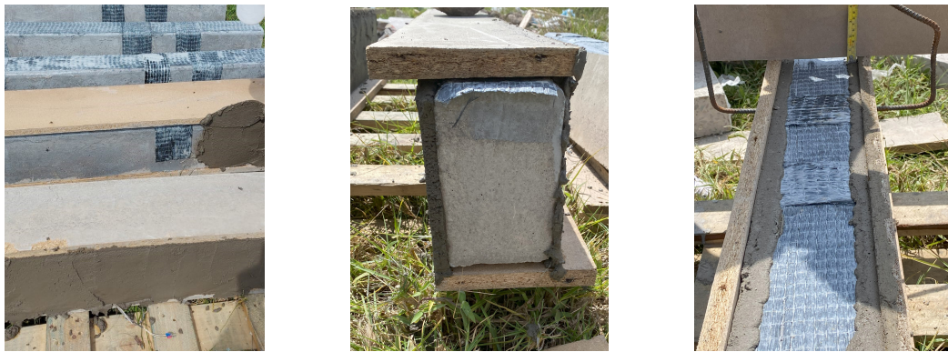
(a) Applying the mortar
