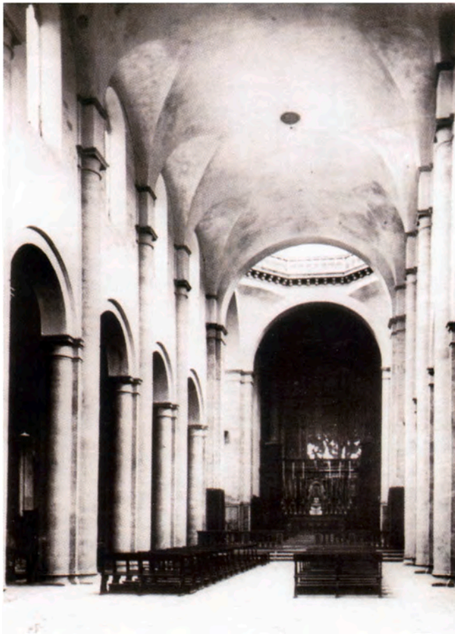
Fig. 2. Period picture, showing the same shot as in the previous picture, representing the condition of the cathedral after the works (1926–1928). The first, glaring evidence is the removal of chains at the arches of the vault in the nave.
