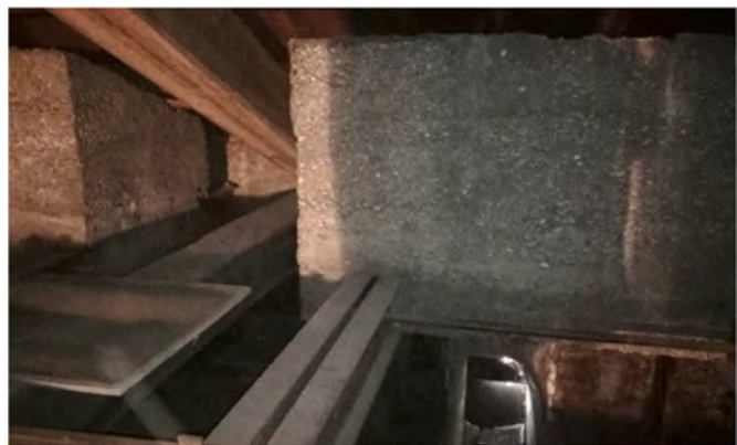
Fig. 5. Concrete blocks and coupled iron supporting beams.
