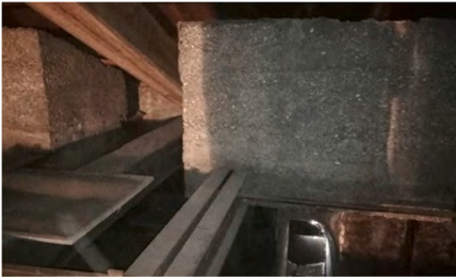
Fig. 5. Concrete blocks and coupled iron supporting beams.
