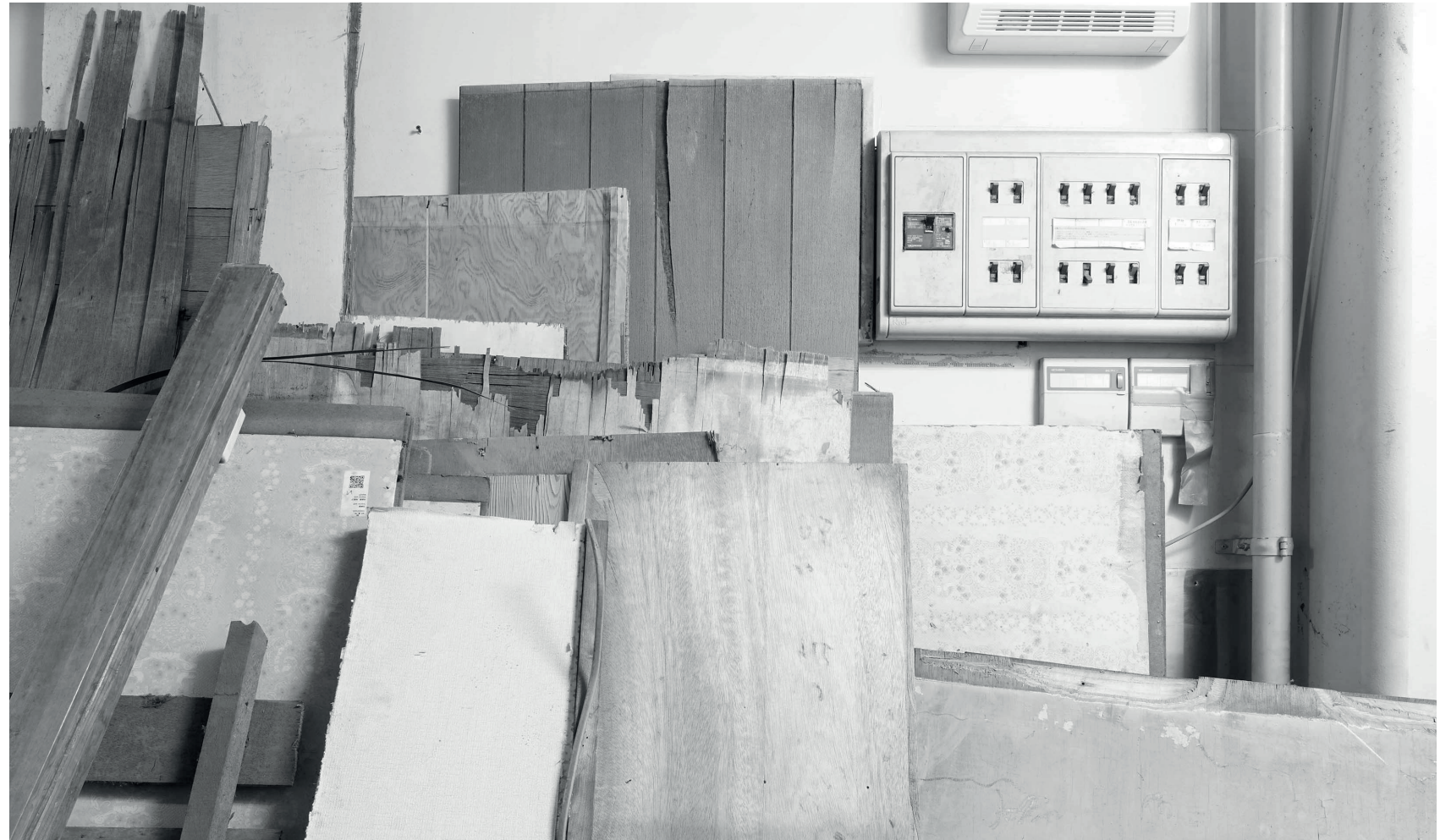
Dismantling Takamizawa House, 2019 ©Jan Vranovský
