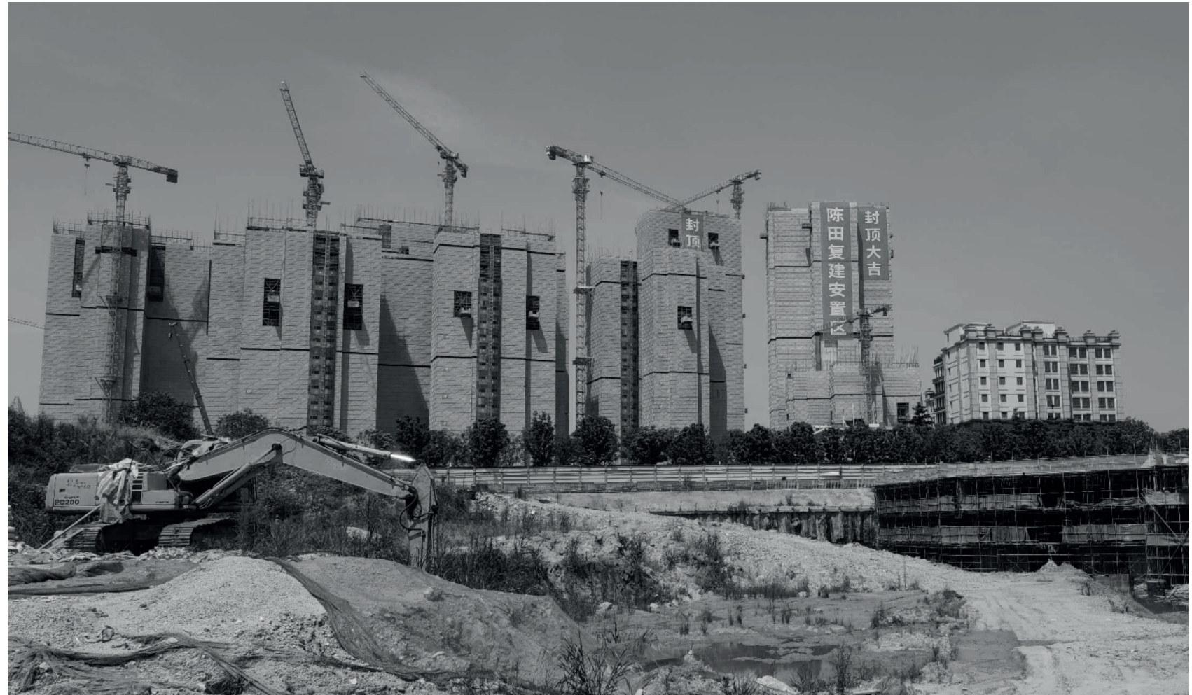
Renovated houses for urban villagers © Shan Jia
