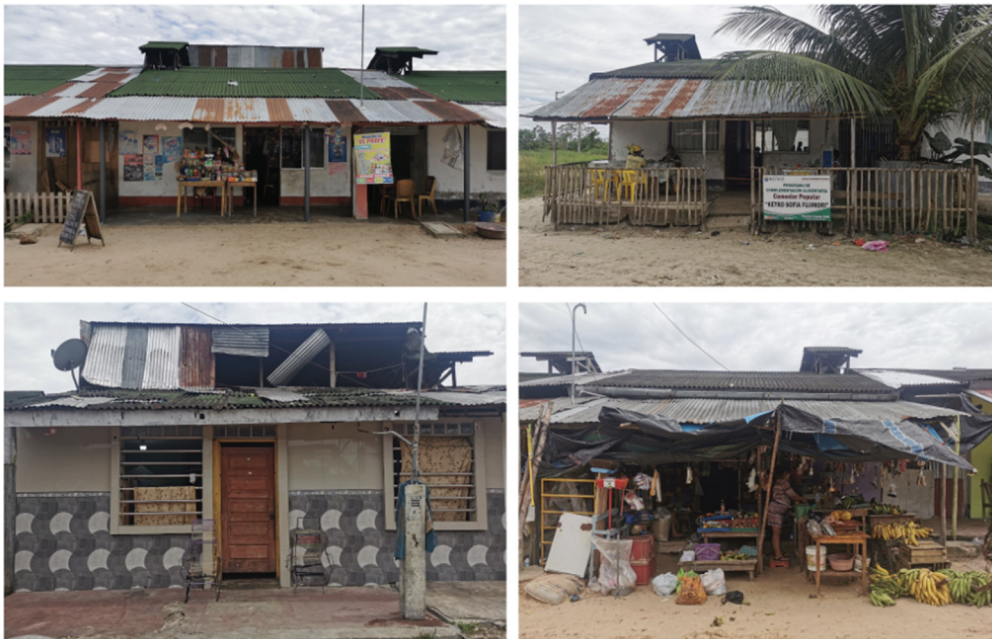
Figure 2. Transformation to houses in Nuevo Belén done by residents. Credits: author, 2022.
