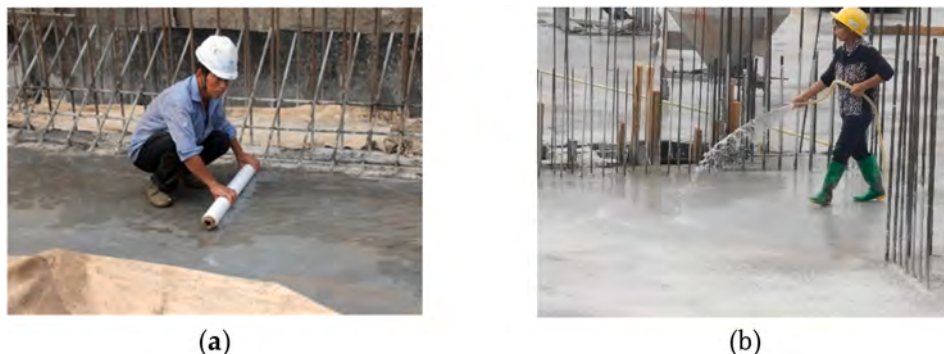
Fig. 1. Concrete curing methods: (a) Plastic film curing; (b) Water spray curing.
