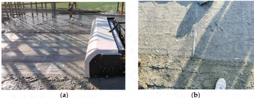
Fig. 16. Comparison of robot and manual curing operation effect: (a) The effect of robot plastic film curing; (b) The effect of manual plastic film curing.
