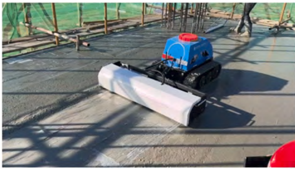
Fig. 15. Robot plastic film curing operation.
