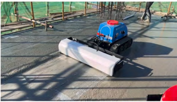
Fig. 15. Robot plastic film curing operation.
