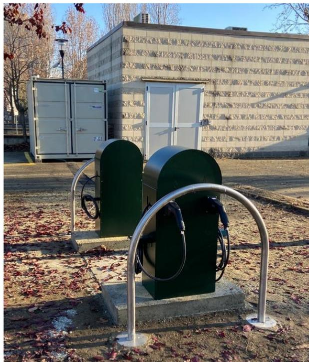
**Figure 3.** Caio Mario substation and low-power chargers inspired by Turin's iconic "Turèt" fountains [30].
