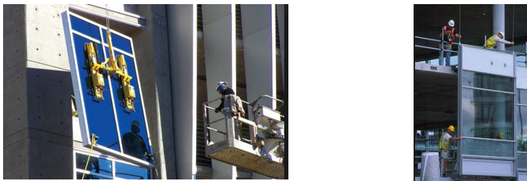
Fig. 1 Installation of traditional non-integrated frame unitised panels for curtain wall systems.
