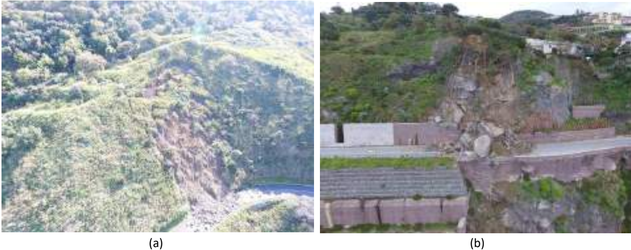
Figure 1 - Landslides events occurred in the municipality of Gioiosa Marea (ME) in March 2016): a) a debris flow on SS113 km 87+060, and b) a rockfall on SS113 km 87+600.
