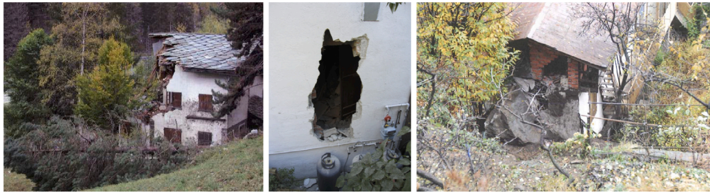
Fig. 3. Damaged buildings due to rockfall events. Photos by courtesy of Autonomous Region of Valle d'Aosta and ARPA Piemonte.
