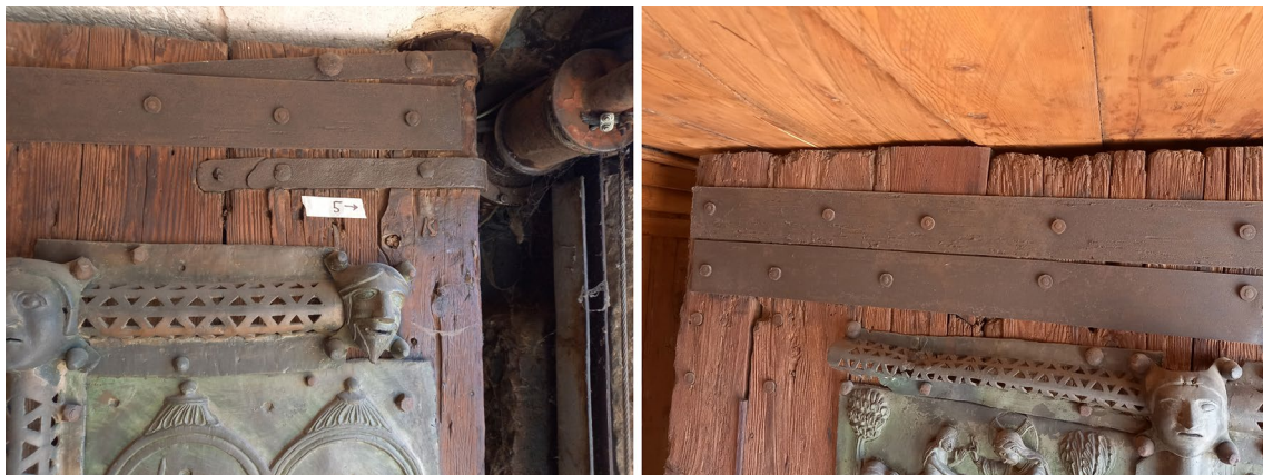
Fig. 14 Details of the wooden door frame. Left. The upper corner of the right wing: you can see the vertical spruce boards and, at the end of the wing, where the arrow points, the board that also serves as the fulcrum. Right: vertical spruce boards and a part restored with pine wood
