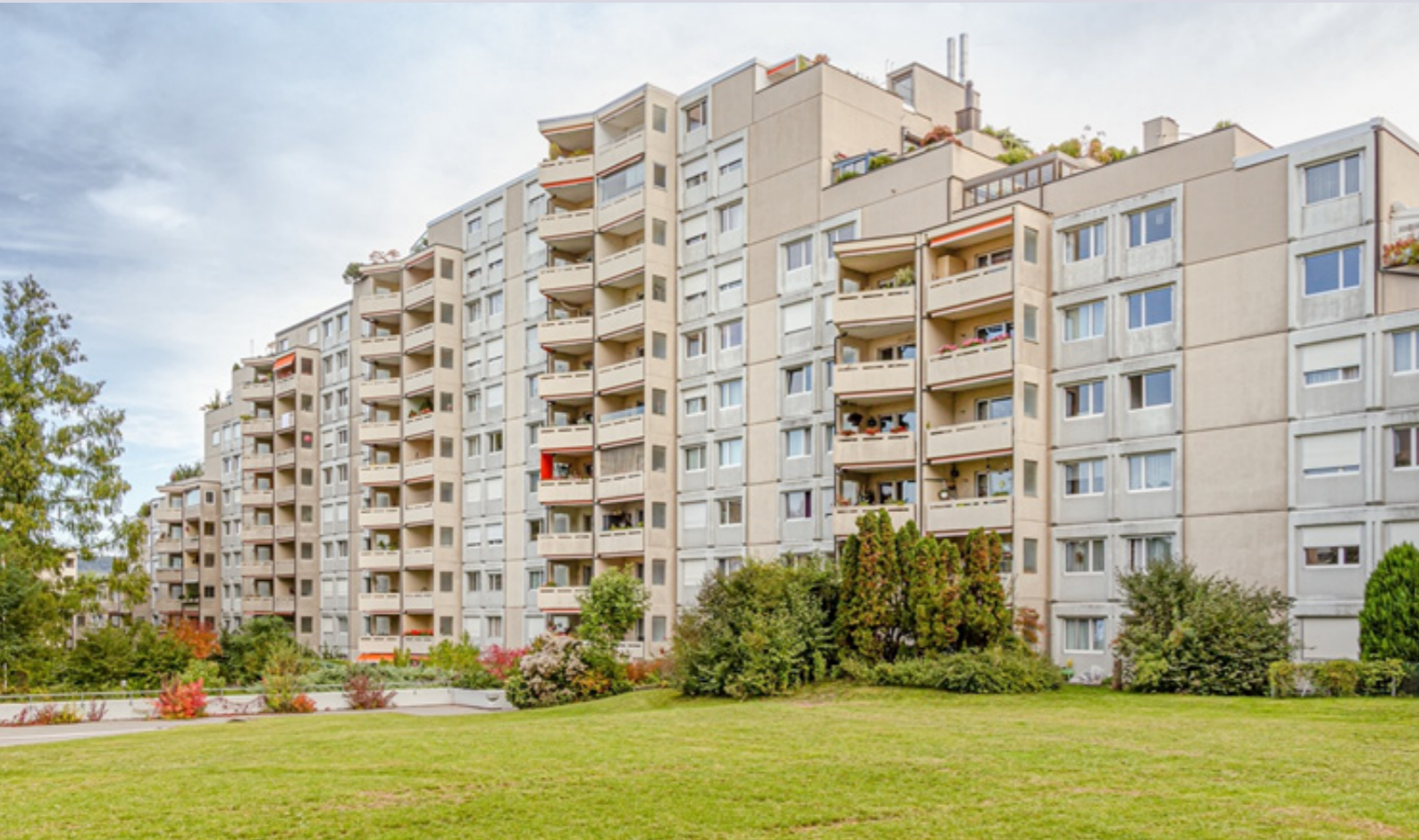
Langgrüt housing estate, Zürich, market-rate rental and condominium apartments, Ernst Göhner AG, 1968–1971 (© photo: Marc Landolt, 2019, Hochschule Luzern – Technik & Architektur)
