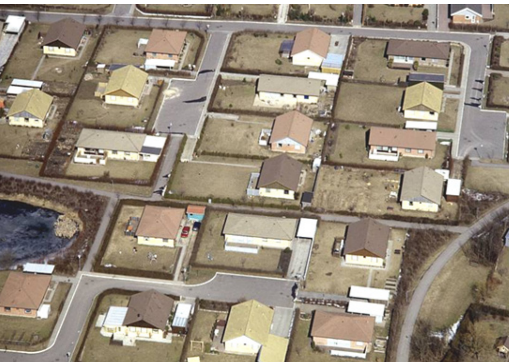
Image of middle class mass housing in Denmark (© photo: Claus Bech-Danielsen, 2004)
