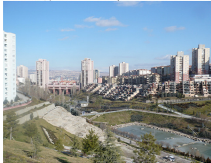
Dikmen Valley Housing Project in Ankara (© Sabah Emlak: Autonomous, 2009; http://mimdap.org/2009/06/dikmen-vadisi-kentsel-donuthum-projesi-iptal-edildi/ )
