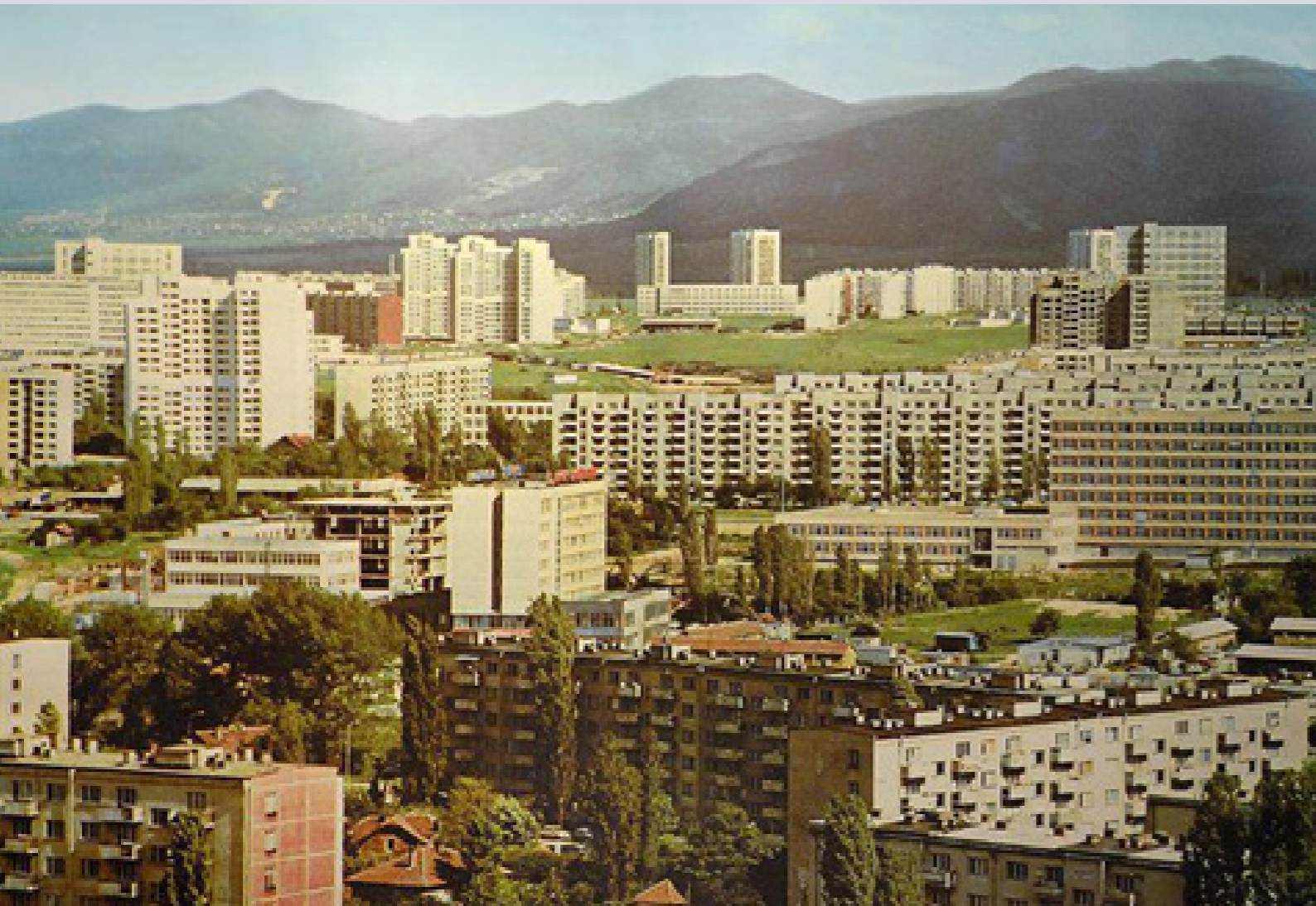
Mladost residential estate in Sofia, built 1980s (© 2023 Брсномех)
