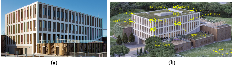
Fig. 1. View of the hybrid timber building (a) and sensor placement (b).
