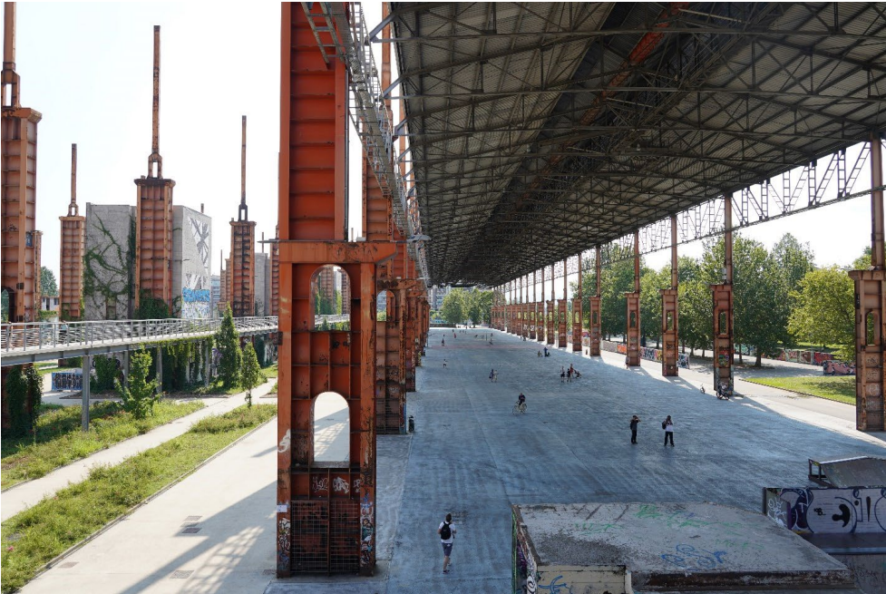
Figure 1) View from South-West of former Vitali's sheds 10 years after the adaptative reuse, designed by Latz and Partners, June 2021, Parco Dora, Turin
