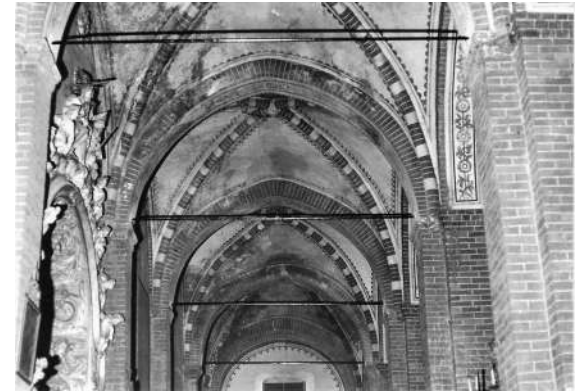
Fig. 2 The chains in the left nave during the restoration yard of 1974-1977 (Parish Historical Archive).
