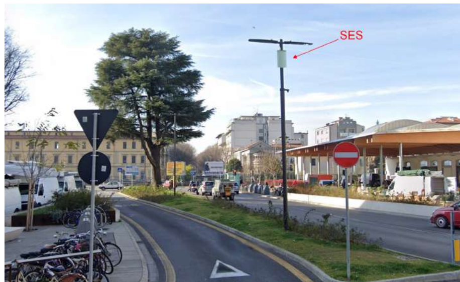
Figure 2. Light pole supporting a curved SES located in a cylindrical radome.
