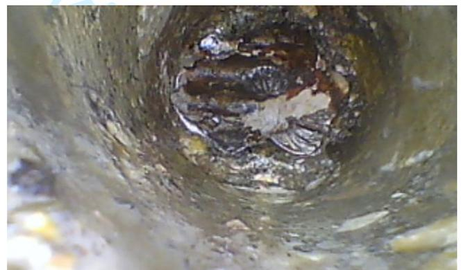
Figure 6 Video-endoscopy to check tendon deterioration.
